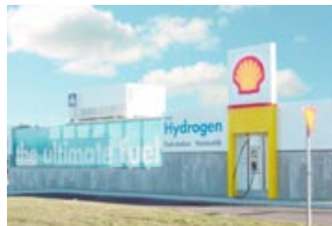
A hydrogen fuelling station in Reykjavik.
