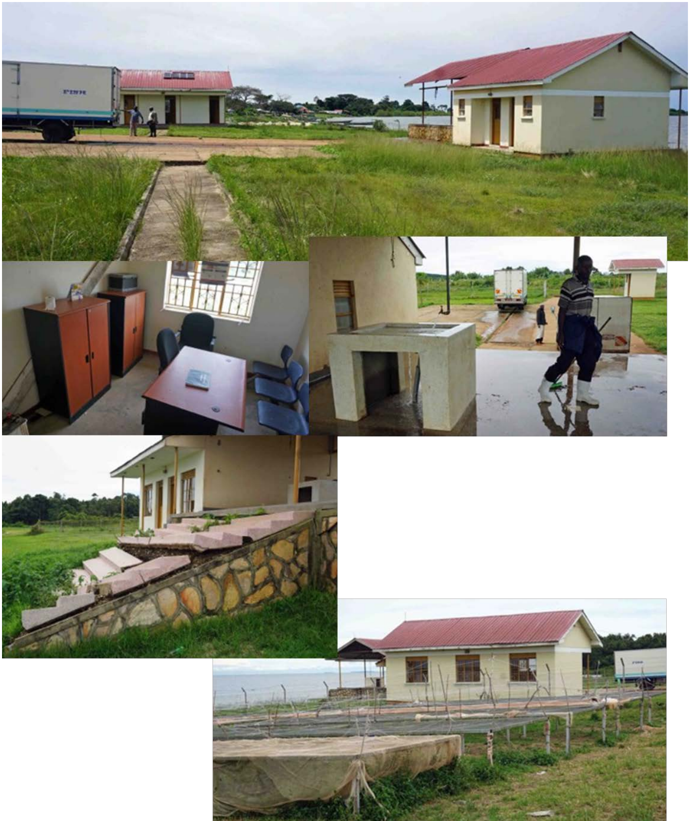
Kyagalanya Fish Landing Site. Nice offices with furniture. Water is present and supplied by Kalangala Infrastructure Services (KIS) through pipeline from Kanasi fish landing site nearby. The stairs to the fish washing stand has been destroyed by flood water and needs to be rebuilt. Fish drying racks not in use at the time of the visit.
