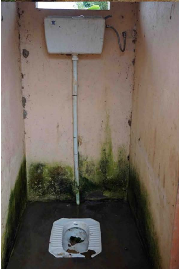
Public toilet in Kasekulo-Ttubi village, not properly cleaned, and with unattractive appearance. Toilet cistern not functioning (considered not appropriate design for rural areas) and no water available for hand washing or toilet flushing.
