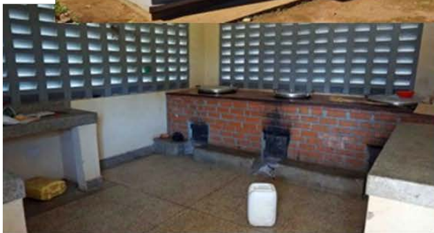
The schools kitchens have appropriate design with own building for firewood and other storage. The tilted air gutters were found to be the best ones, as the design prevents the rain from entering. The energy-saving stoves has reduced the firewood use to 1/3 of previous level. From top left: Bufumira PS, Kibanga PS, Mulabaka (w/headteacher), Bwendero PS (3 photos).
