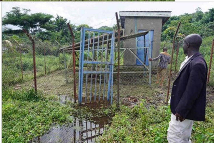
Kachungwa Fish Landing Site. The fish drying racks in use in the village (Kachanga), except for the rusty ones on the right side. Water supply pump house with difficult access due to swampy area around. Solar panels need cleaning.
