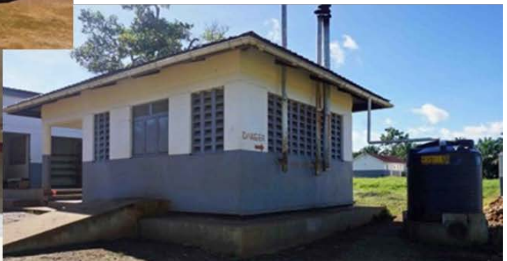
The schools kitchens have appropriate design with own building for firewood and other storage. The tilted air gutters were found to be the best ones, as the design prevents the rain from entering. The energy-saving stoves has reduced the firewood use to 1/3 of previous level. From top left: Bufumira PS, Kibanga PS, Mulabaka (w/headteacher), Bwendero PS (3 photos).
