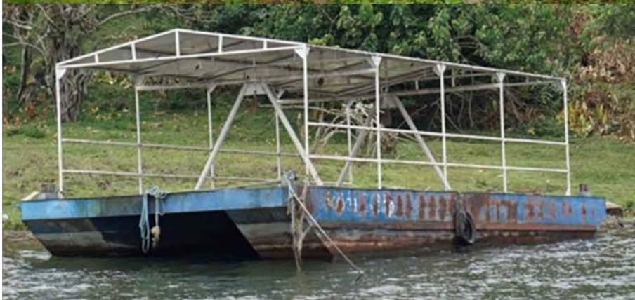
Kachungwa Fish Landing Site. Overview photo: village to the right and landing site to the left of the forest (with water supply house on very left). Site obviously not much used to judge from appearance. All buildings were locked as the Sub-County Fisheries Officer had gone away with the key! Building show signs of deterioration (a lot of birds' nests and rusty roof beams). The floating barge, no more in use (not suitable in rough weather).
