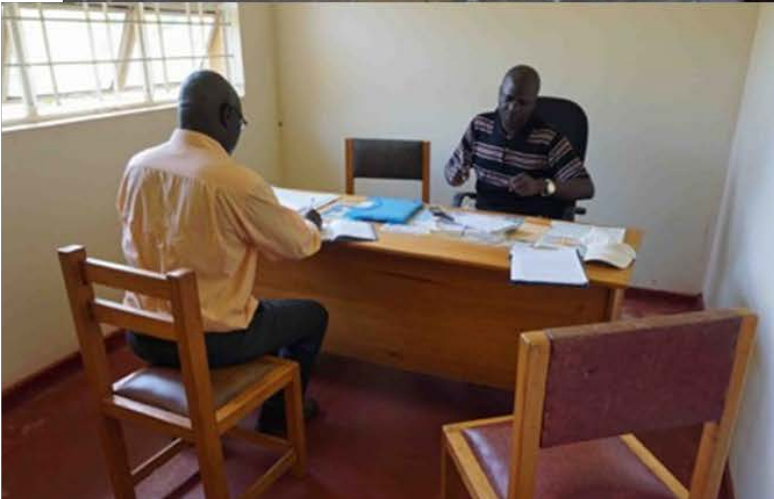
Bubeke Sub-County Office. Nice offices with good furniture. The building shows signs of serious deterioration. The Sub-County claimed to have very little (read: no) money to undertake proper O&M.
